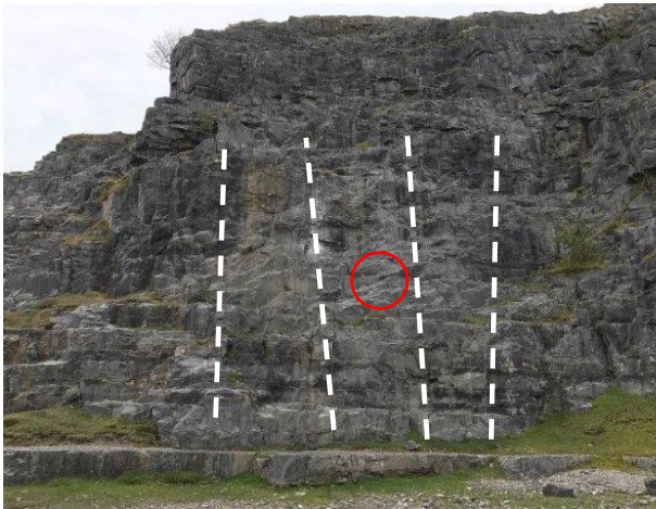
Be aware of metal pipe, circled
